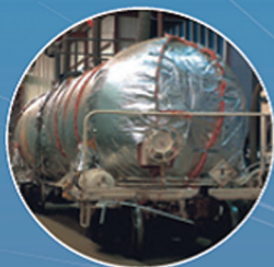
Tank Car Repair
